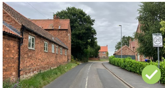
Figure 33: New development is responsive to its setting by providing a termination to this view along the street. Red brick and clay pantiles have been used to complement the character of existing farm-buildings (to the left).
