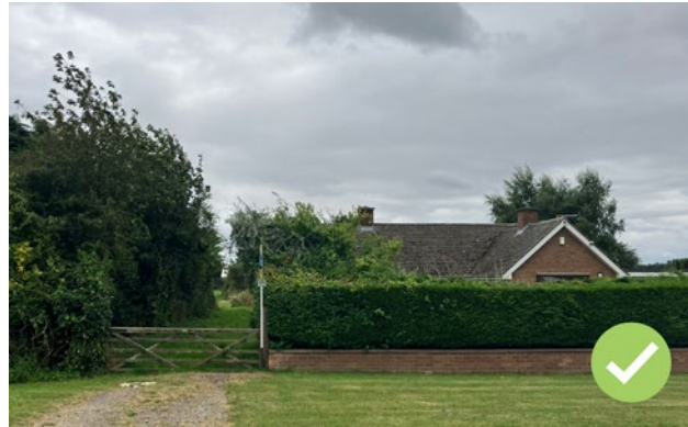
Figure 23: Hedgerows and mature planting help to screen development from the street, enhancing the rural setting.
