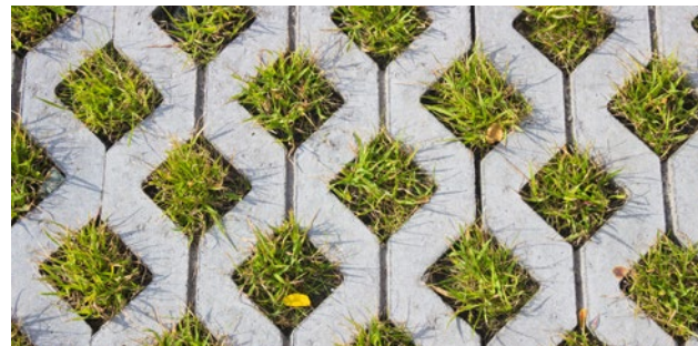
Figure 66: Permeable paving solutions such as grasscrete should be used on-plot wherever possible.
